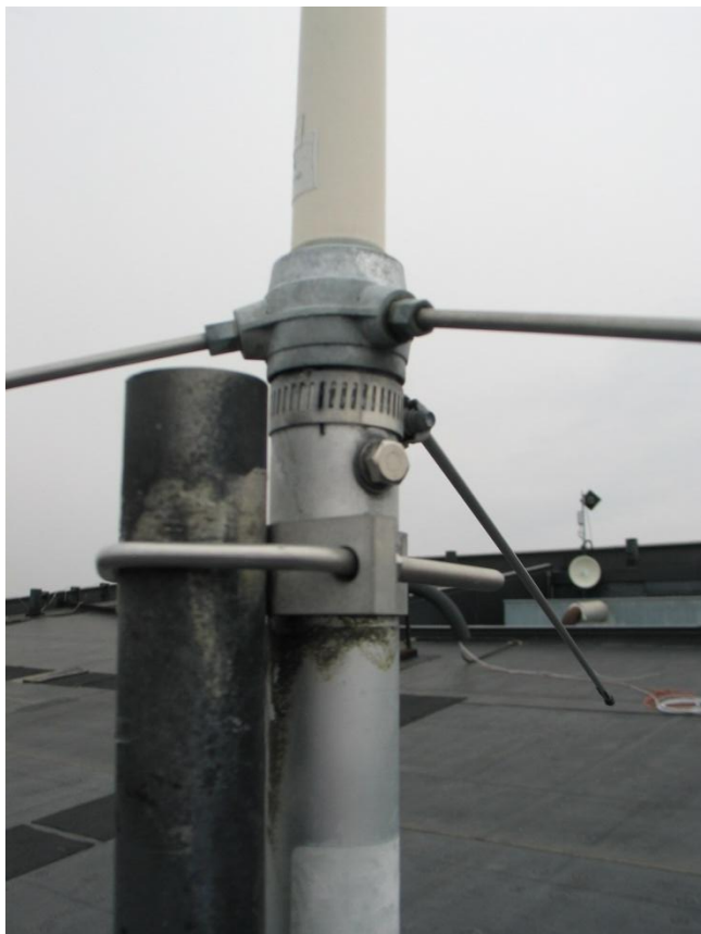
Figure 4 - The hex bolt after we replaced it
